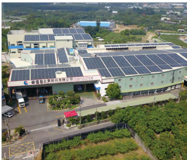
SCF's factory is now equipped with fully installed solar panels, capable of generating 1,500,000 kWh of electricity annually, equivalent to reducing carbon emissions by 750 metric tons of CO2e each year. (Photo provided by Shuenn Chang Fa)
